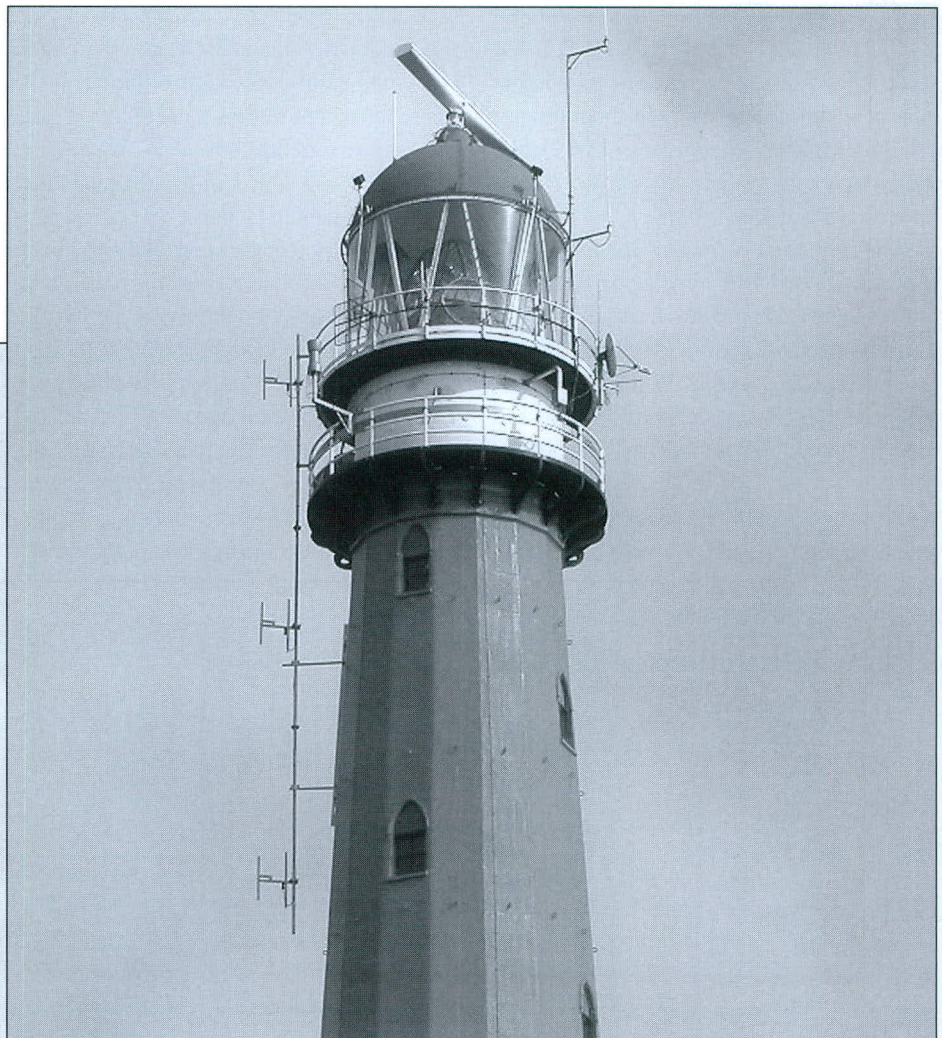
The new steel lantern installed on Lange Jaap in 1992. Note the diagonal astragals and the large array of antennas. The lights above the glass panels illuminate the dome at night to prevent bird strikes. Photo by the author.
