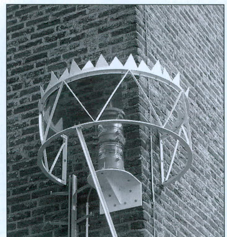
Schulpengat Light is a beacon on the corner of the Channel Traffic Control Building beside the fort. It shines a continuous red sector warning ships away from the Noordhaaks sand bar. Note the serious bird "discourager." Photo by the author.
