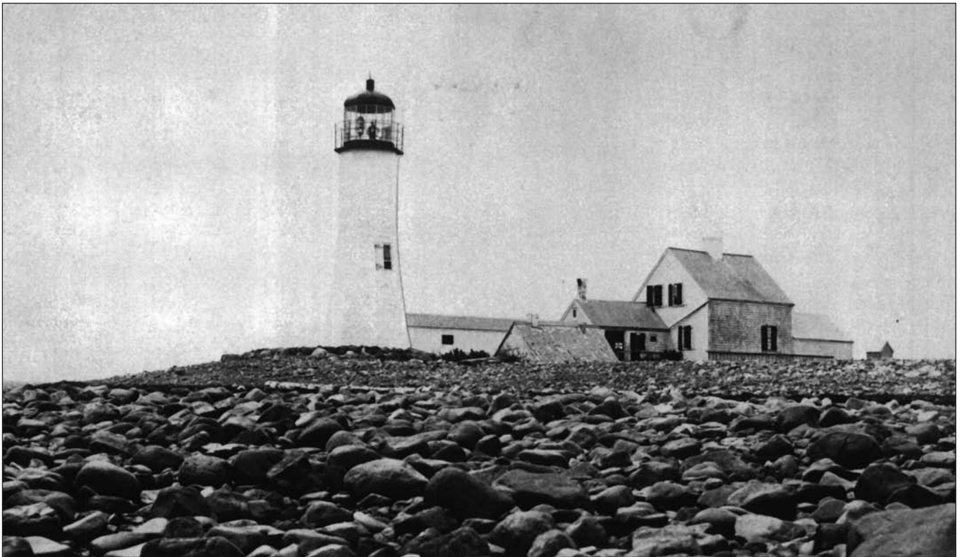
Scituate Lighthouse, circa 1857. Note the keeper in the lantern room and that the optic is off center. By this date a Fresnel lens has been installed. USLHS archive photo.
