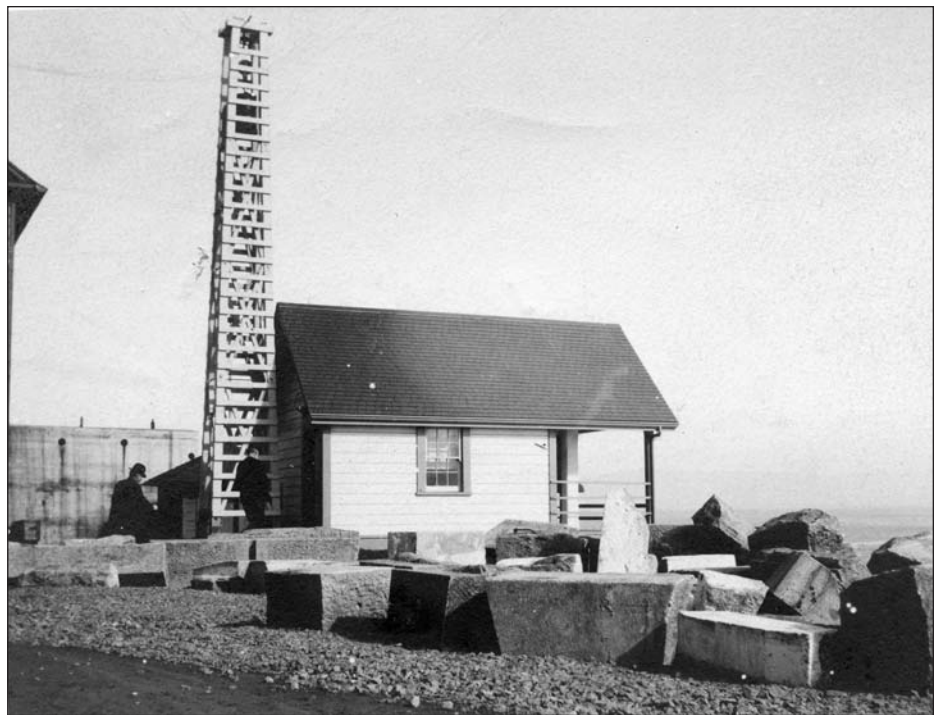
Because the weight cables of the first Alcatraz fog bell (below) kept falling, a second house with a weight tower at the rear (above) was constructed. USLHS archives.
