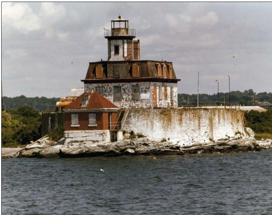
The Rose Island (Rhode Island) Lighthouse, in 1985, was deserted and left to the elements before preservation efforts brought it back (bottom photo). USLHS archive photos.
