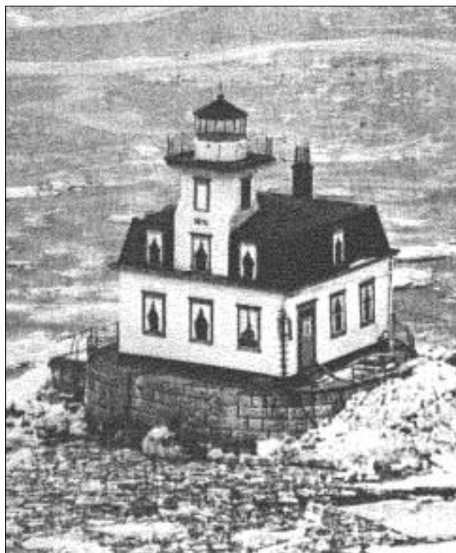
Esopus Meadows Lighthouse surrounded by ice in the middle of the Hudson River in New York. To discourage vandals, the Coast Guard painted curtains on the boarded-up windows. One also has a cat painted in and another a flower pot.
