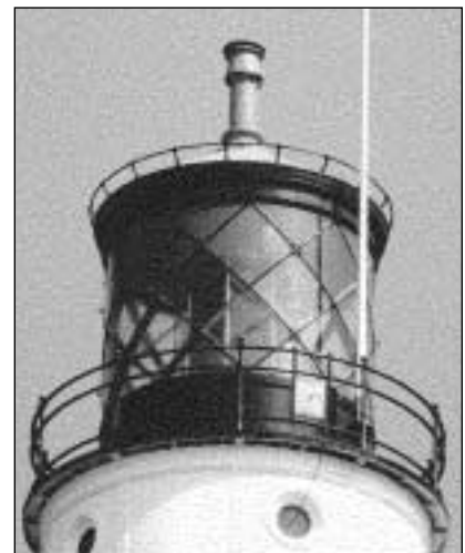
A lantern room with a fixed first order Fresnel lens.
