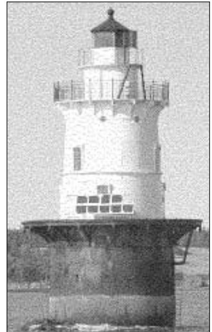
A round caisson, or "sparkplug" lighthouse
