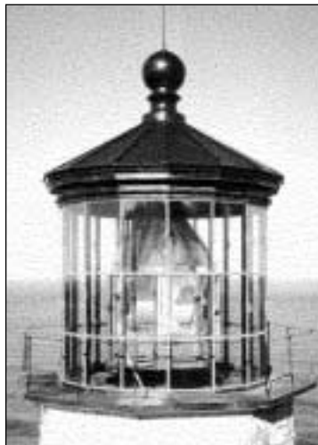
A lantern room with a fixed first order Fresnel lens.
